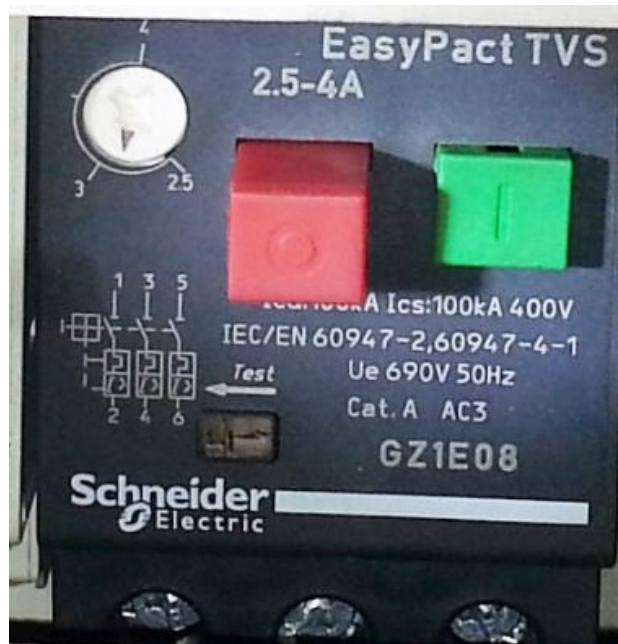
TRIP condition – Red plunger in pressed condition
