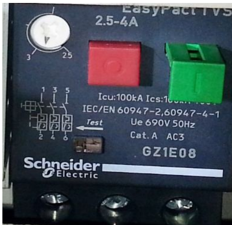
TRIP condition – Red plunger in pressed condition
